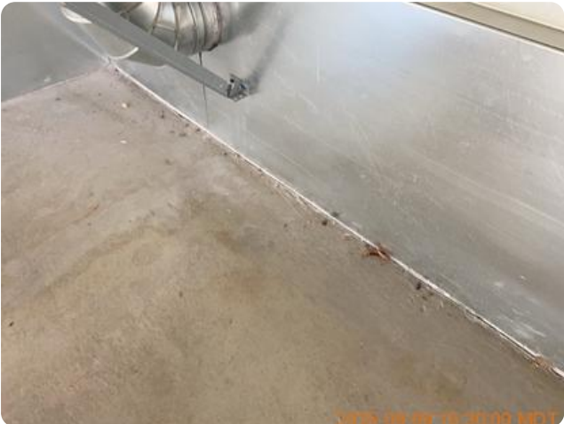
Driveway/Floor 2025-08-06 15:30:00 40.42186951033655, -111.8638431834066 View Image
